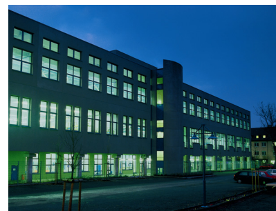
OBE Germany - 15.000m 2 production area
